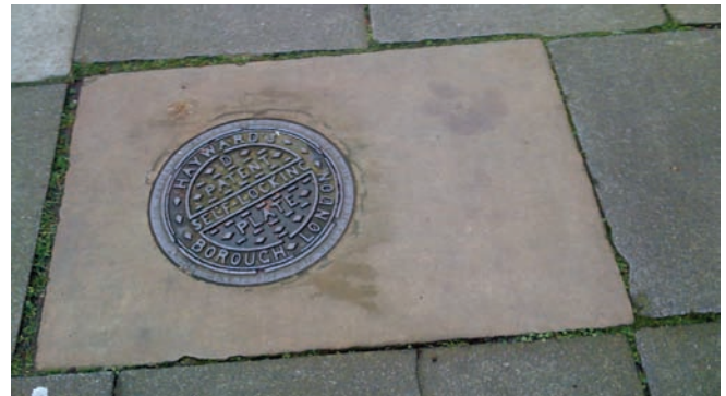
There was probably little wrong with the rest of this stone pavement (at Gloucester Circus, Greenwich) but it was replaced, leaving only the pavers with coal-holes inset
